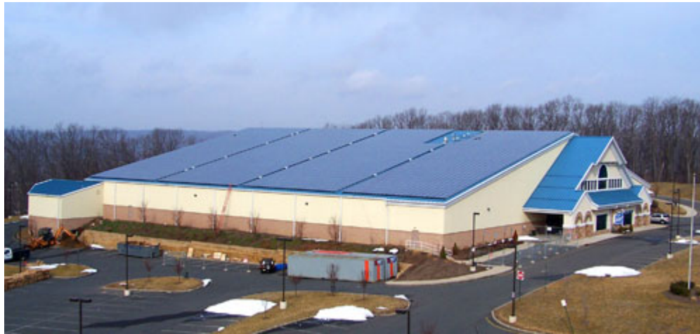
Its Sharp solar electric system reduces energy consumption at the Aspen Ice rink by more than half.
