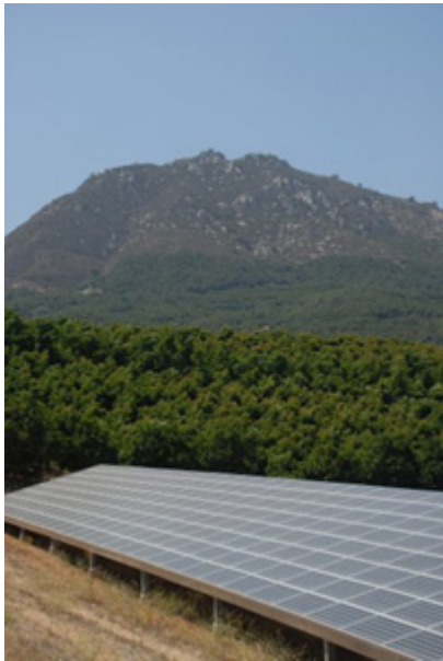
Covering two acres of a five-acre plot, the solar installation consists of 6,310 industrial-grade Sharp solar modules.
