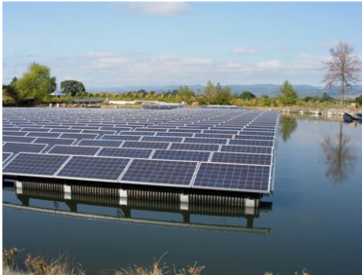
Floating the solar panels on the vineyard's irrigation pond saves valuable vineyard acreage
